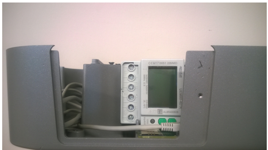
Fig. 11 G7 station with installed MID meter
